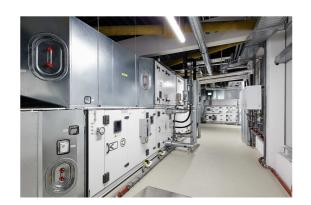
Nine X-CUBE air handling units provide ventilation to the new building at the expanded engelbert strauss company site.
