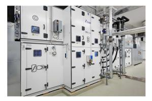
As a special feature one of the air handling units was designed to be built around a pillar – which could not be moved.
